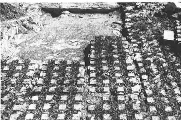
FIGURE 5 Precast studded-slab construction.
