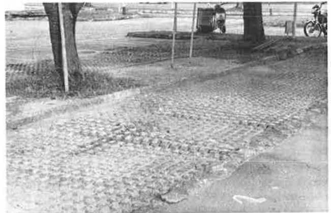
FIGURE 3 Studded-concrete-slab pavement construction for parking areas.
