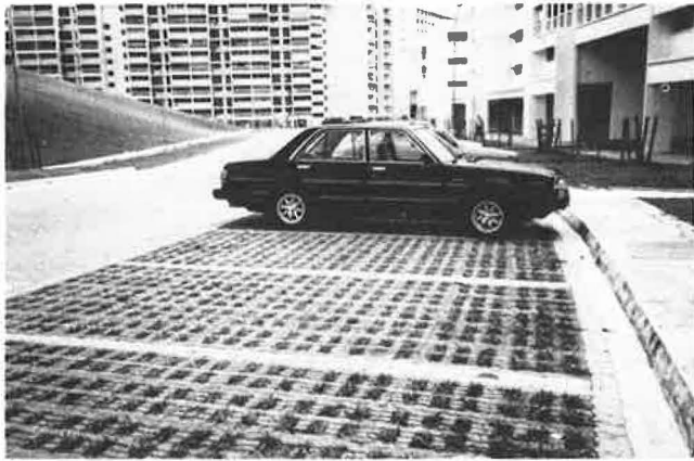
FIGURE 11 Interlocking-perforated-block pavement.
