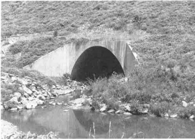
FIGURE 9 Downstream end of Little Bull Creek arch culvert.
