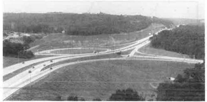
FIGURE 3 Bull Creek Road Interchange of the Allegheny Valley Expressway.
