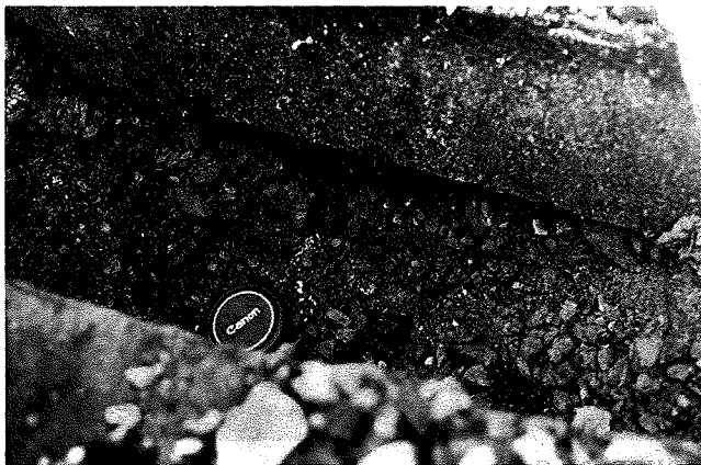
FIGURE 6 Mile 65.0, Mountain Subdivision.
