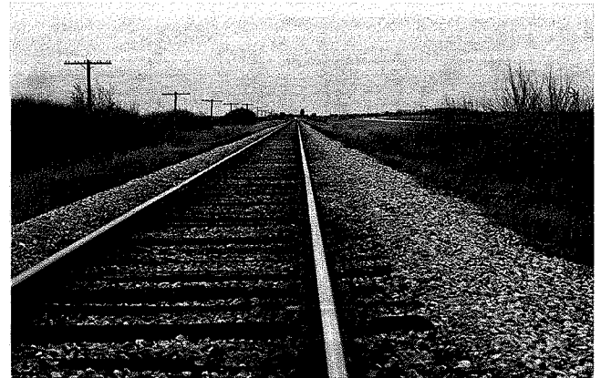
FIGURE 12 Good performance of ballast.
