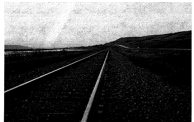
FIGURE 13 Poor performance of ballast.
