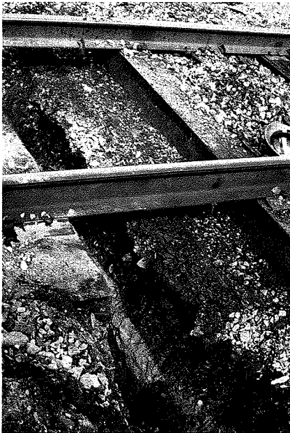
FIGURE 10 Mile 110.4, Ignace Subdivision.
