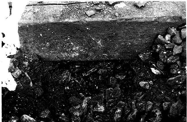
FIGURE 8 Mile 52.2, Mountain Subdivision.
