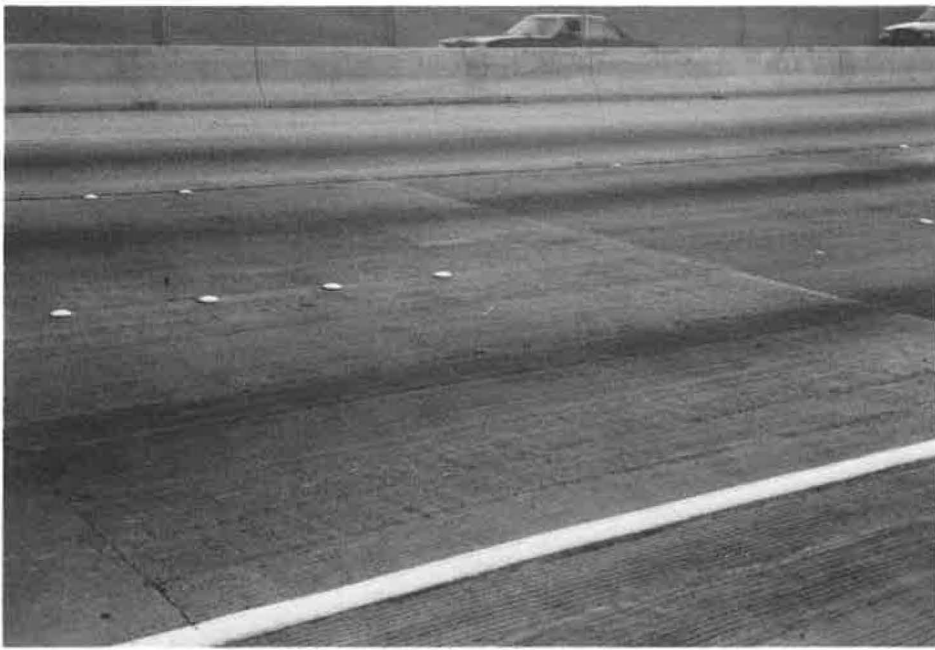
FIGURE 10 Repair of concrete.
