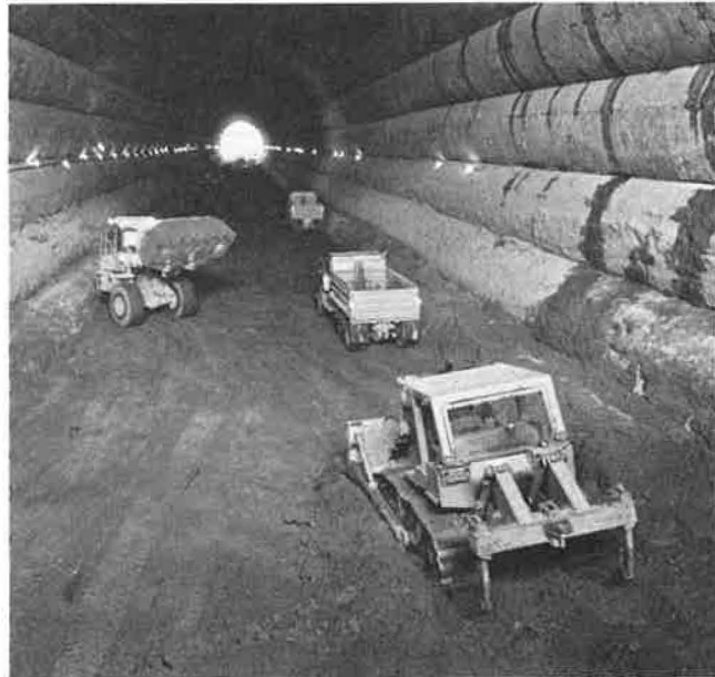
FIGURE 1 Tunnel mass excavation near completion (Richard S. Heyza/Seattle Times).
