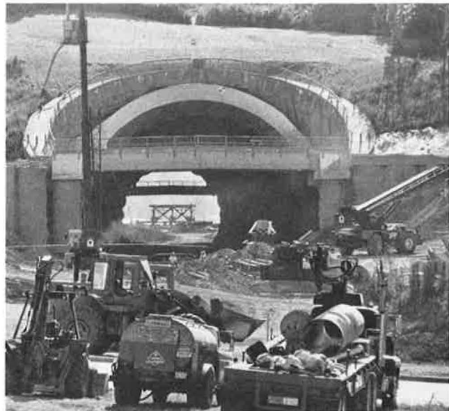
FIGURE 10 View from west through the completed tunnel (Ralph Radford/Valley Newspapers).
