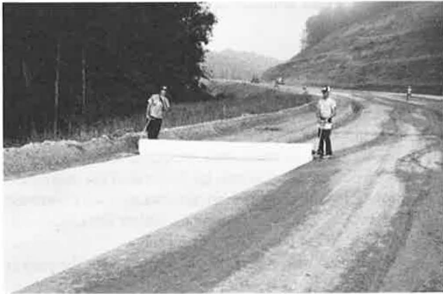
FIGURE 5 Geotextile filter placement.
