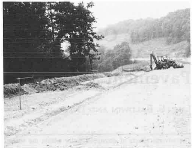
FIGURE 3 Cutting of the underdrain trenches.
