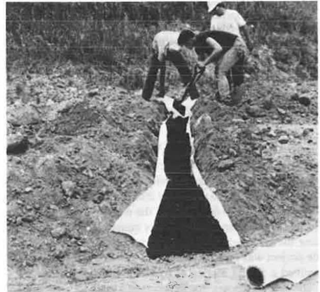
FIGURE 4 Installation of the aggregate-filled fabric underdrains.
