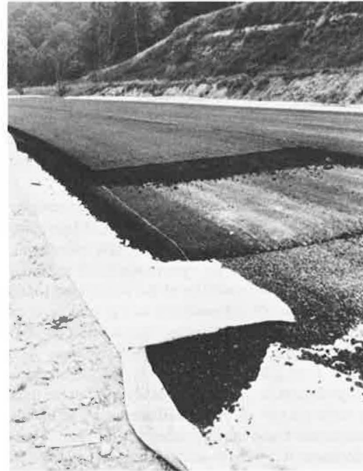
FIGURE 7 Cross section of pavement under construction.
