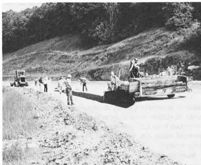
FIGURE 6 Filling of the "V" ditch with free-draining base.
