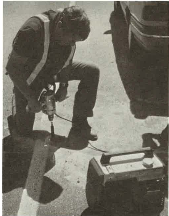
FIGURE 11 Drilling into the edg drain.
