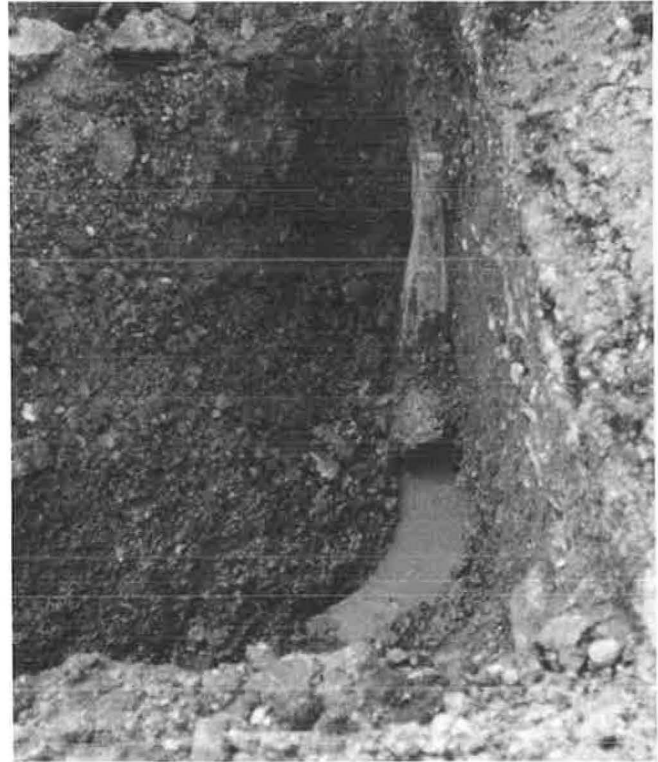
FIGURE 15 Outlet pipe removed.
