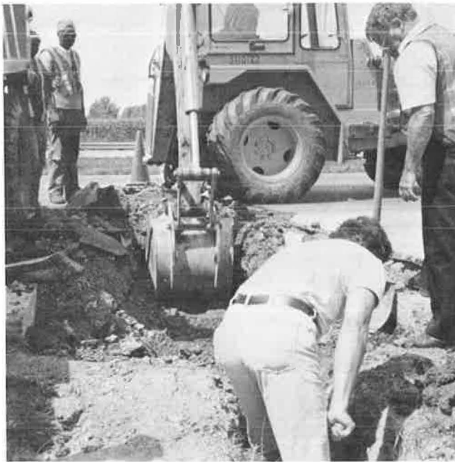
FIGURE 14 Digging up an outlet.
