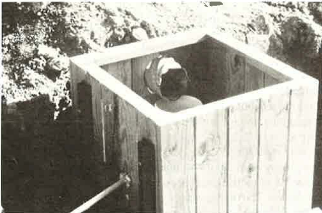
FIGURE 8 Tipping bucket enclosure.
