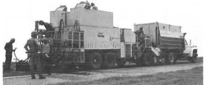
FIGURE 1 Microsurfacing laydown machine with truck.
