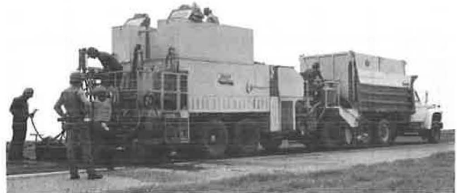
FIGURE 1 Microsurfacing laydown machine with truck.
