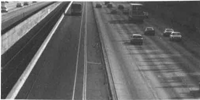
FIGURE 2 HOVL separated from regular lanes by a wide, traversable buffer (center).
