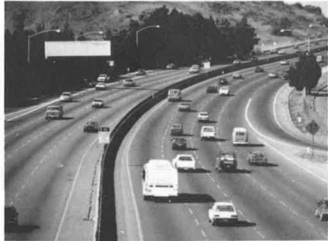
FIGURE 4 HOVL with unrestricted access. In this case, the HOVL is marked by signage.
