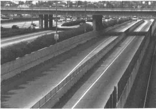
FIGURE 1 Physically separated HOVL. Barrier is visible at left center, with westbound HOVL immediately to the right and the eastbound HOVL at far right.
