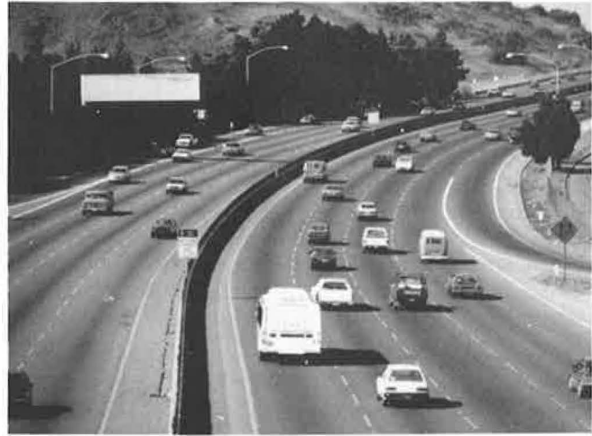
FIGURE 4 HOVL with unrestricted access. In this case, the HOVL is marked by signage.
