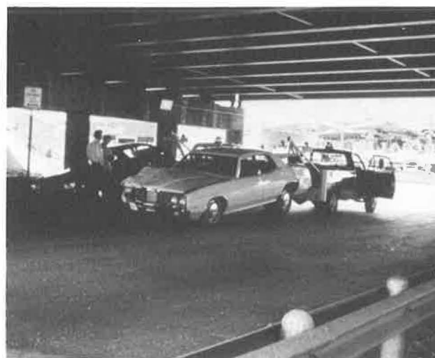
FIGURE 1 AIS under bridge structure.
