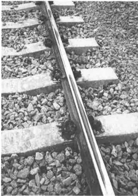
FIGURE 5 General view of reprofiled rail.
