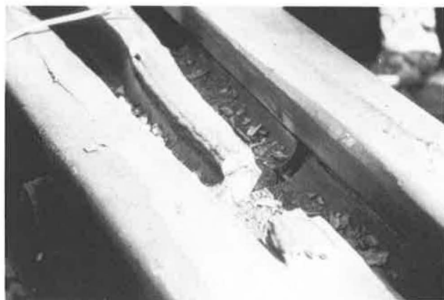
FIGURE 2 Crossing nose requiring repair welding.
