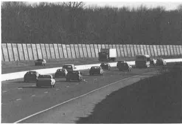
FIGURE 4 Separate post and panel barrier, tilted 10 degrees.
