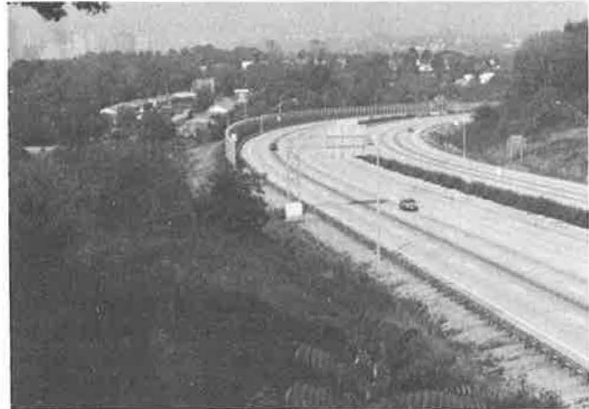
FIGURE 1 Noise barrier, Interstate 471, Campbell County, Kentucky.
