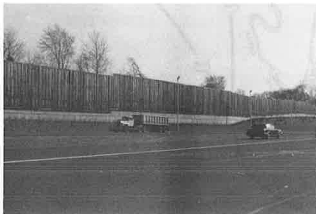
FIGURE 8 Wooden barrier supported by double wall along I-295/195.
