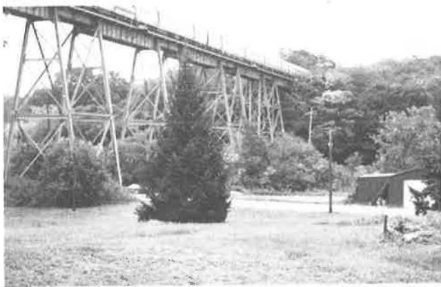
FIGURE 2 View of Manhasset Viaduct.
