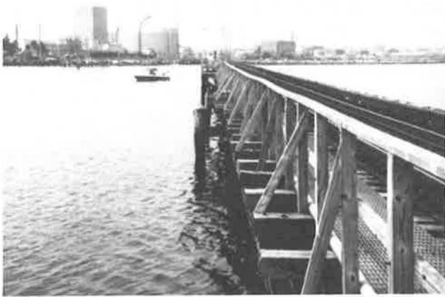
FIGURE 4 Reynolds Channel timber trestle.
