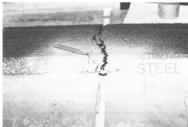
FIGURE 7 Tested steel-compacted slab.
