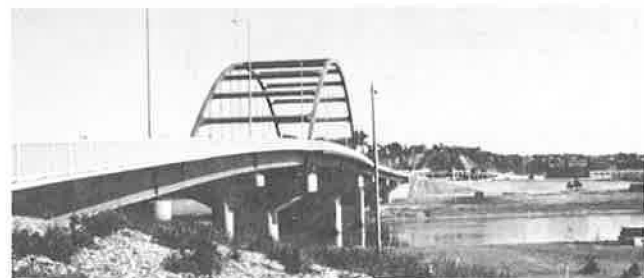
FIGURE 1 Siouxland Bridge at Sioux City, Iowa.
