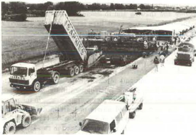
FIGURE 4 Complete paving plant train.
