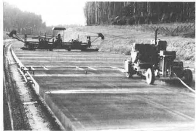
FIGURE 10 Cutting transverse and longitudinal contraction joints with saws.
