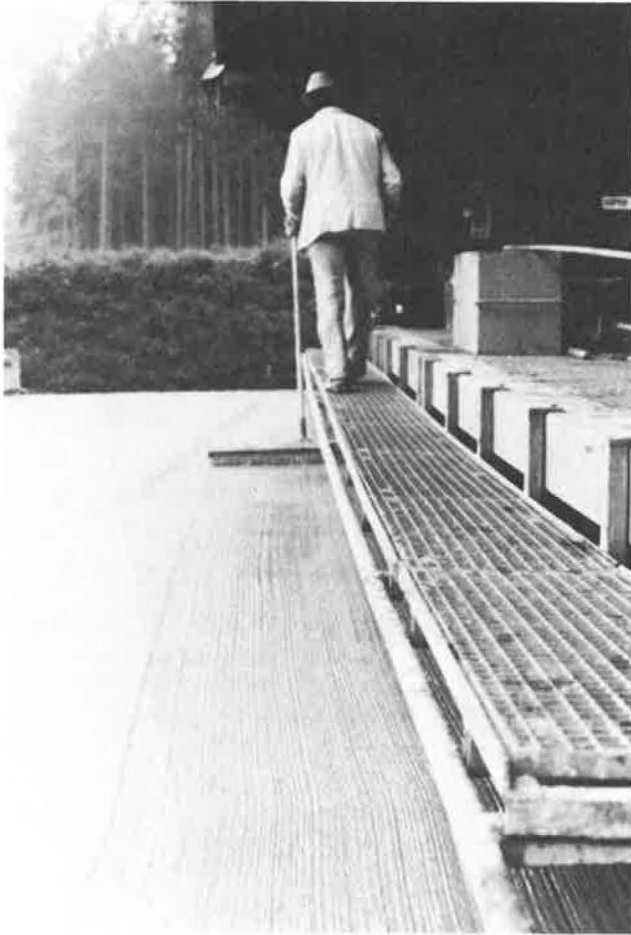
FIGURE 8 Broom finishing.
