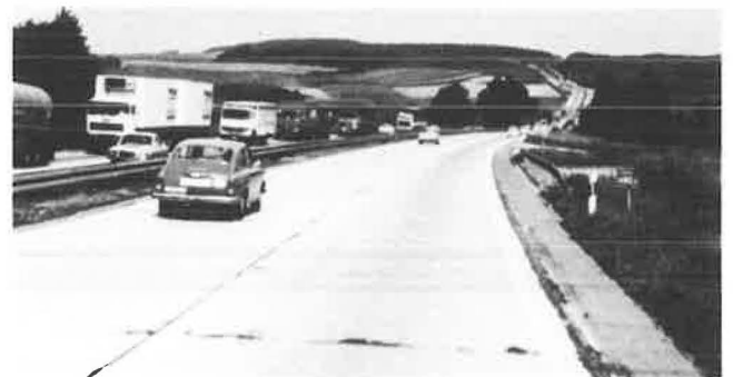
FIGURE 1 Autobahn with two lanes in one direction.
