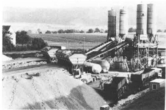
FIGURE 3 Mixing plant for a concrete pavement construction site.
