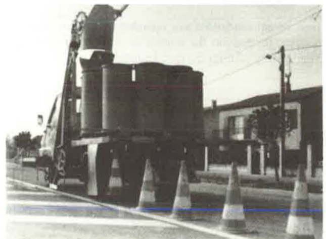
FIGURE 1 Cone dispenser placing cones; their spacing is adjustable.
