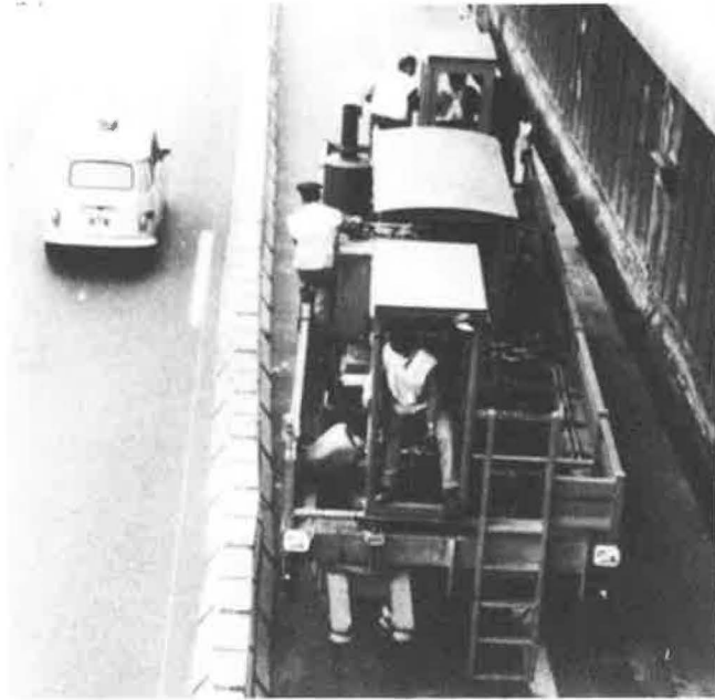
FIGURE 3 Mobile lane separator laying first line of blocks in place.
