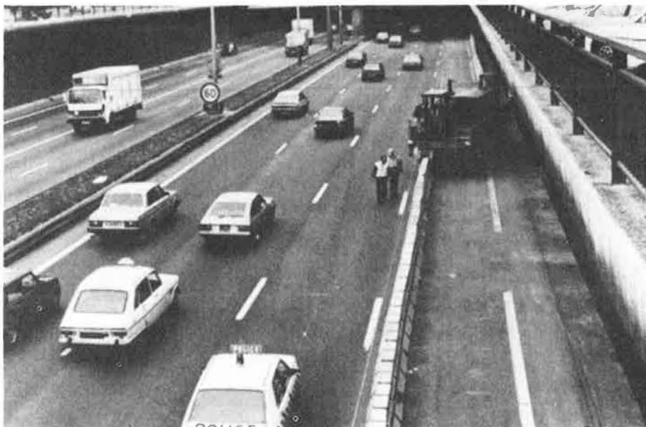
FIGURE 9 Paris exit of Autoroute A1, July-August 1984.
