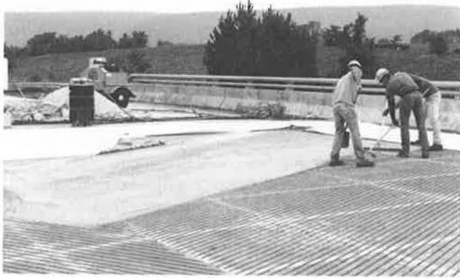
FIGURE 7 Groove-filling operation.
