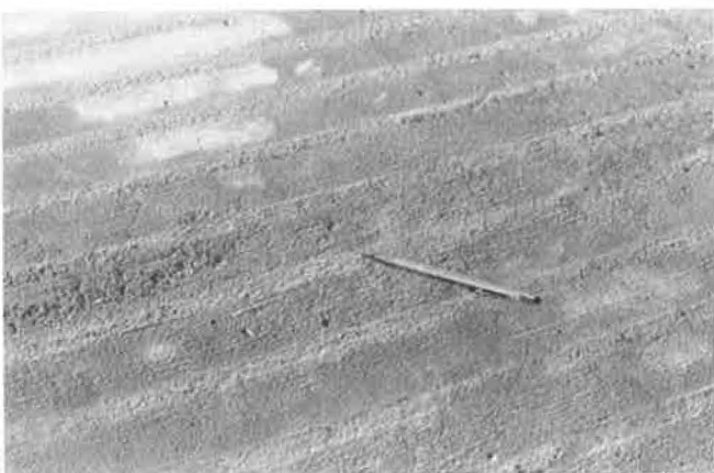
FIGURE 8 Deck surface 1 day after groove filling.
