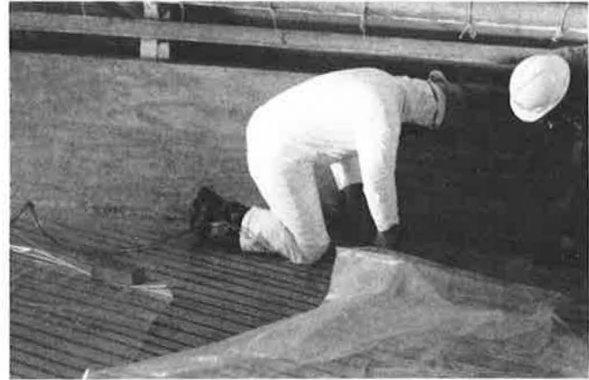
FIGURE 5 Two-man crew filling individual grooves.
