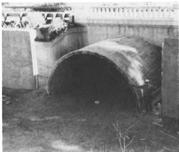
FIGURE 11 San Martinez Grande: three precast units in place.
