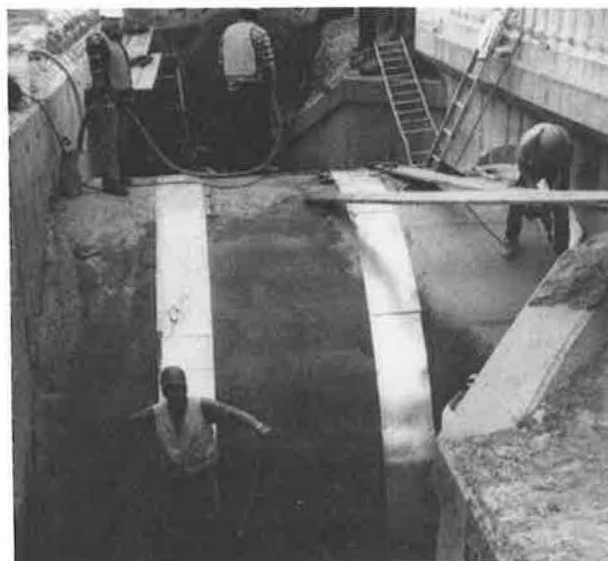
FIGURE 12 San Martinez Grande: backfilling precast units.
