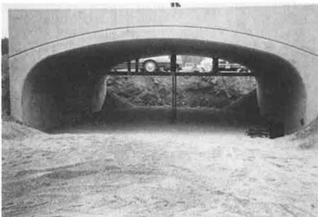
FIGURE 5 Box-arch culvert load test, August 1986.
