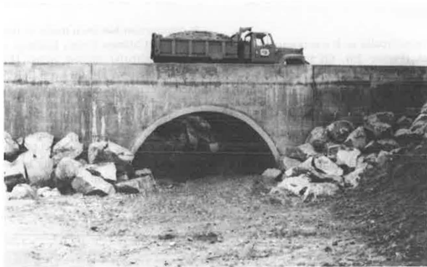
FIGURE 15 Static live load test.
