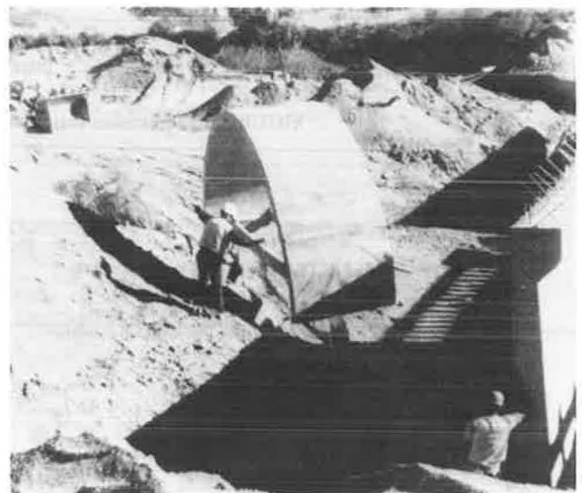
FIGURE 10 San Martinez Grande: lifting precast unit.
