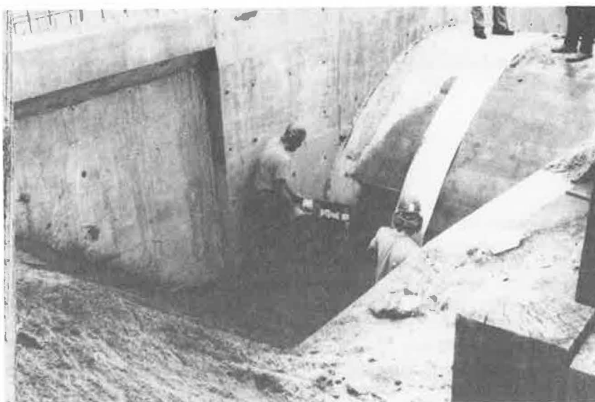
FIGURE 13 San Martinez Grande: compaction with portable tampers.
