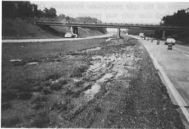
FIGURE 5 Tufa precipitate at edge of shoulder.
