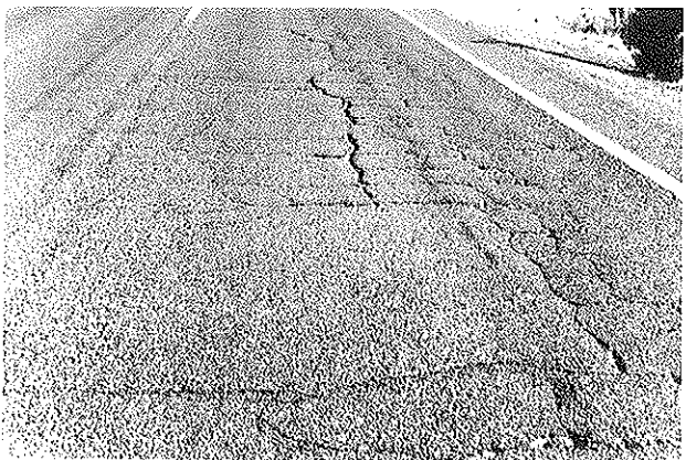
FIGURE 13 Typical cracking, test segment no. 13, SAM (age 48 months).
