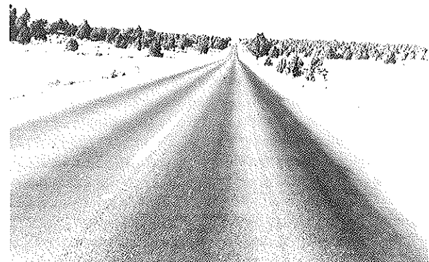
FIGURE 10 Typical wheel track bleeding, test segments 11 and 12, double SAM (age 48 months).
