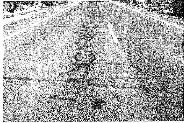
FIGURE 8 Typical raveling, test segments 7 and 8, 0.15 and 0.20 ft conventional DGAC (age 48 months).
