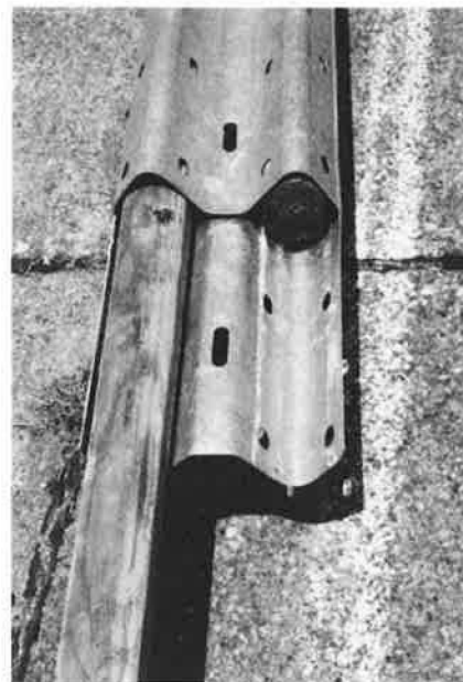
FIGURE 9 Wood inserts for tubular W-beam.
