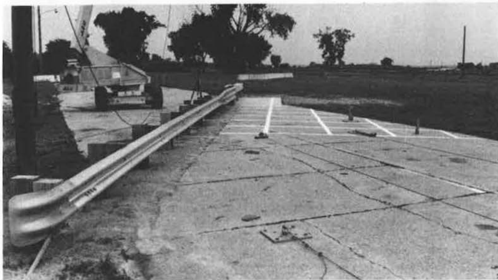
FIGURE 4 Photographs of approach guardrail installation.
