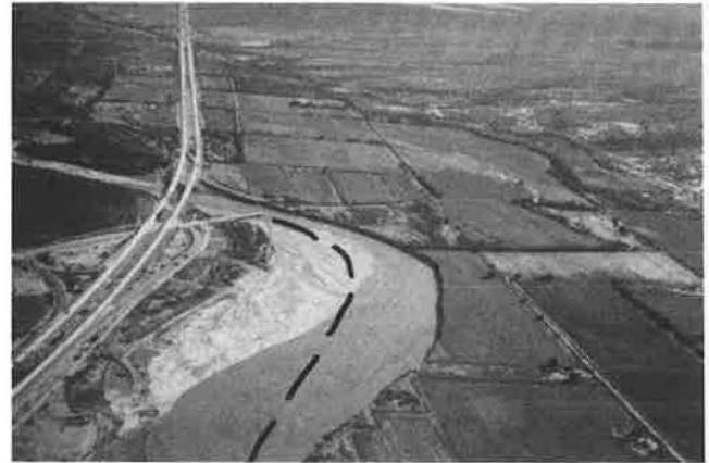
FIGURE 8 View looking south and upstream at the Santa Cruz River at Interstate 19 on October 3, 1983. The right bank abutment of the northbound lane failed and the left bank abutment of the bridge to the right of Interstate 19 was destroyed during flooding on October 1 and 2. The dashed line approximately represents the location of the left bank of the entrenched channel before the flood.
