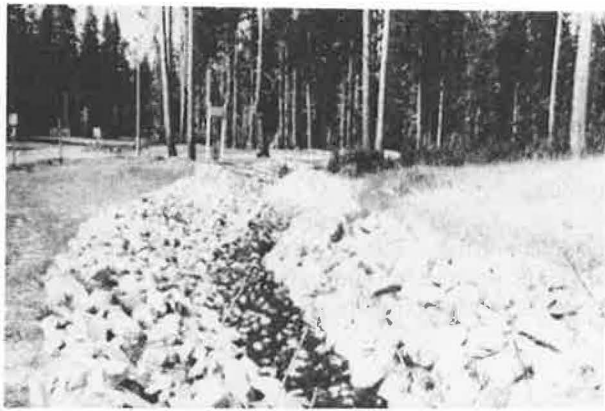
FIGURE 5 (Top) Old channel basin. (Bottom) Realigned section of East Benwood Creek.
