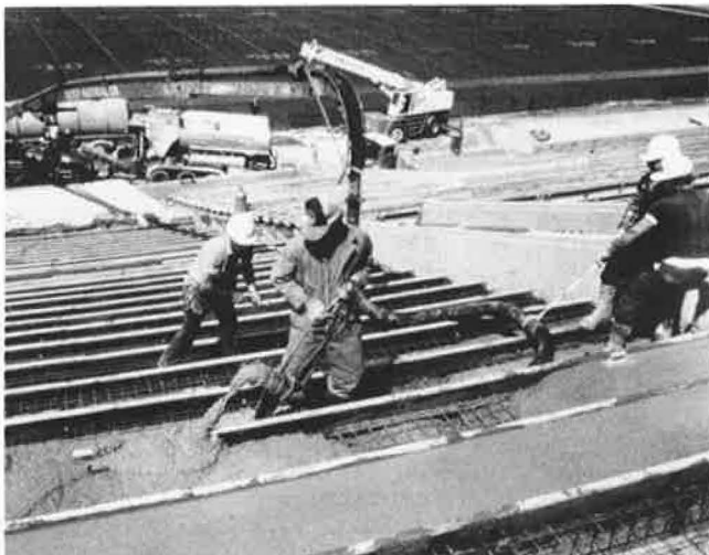
FIGURE 9 Placement by pump.
