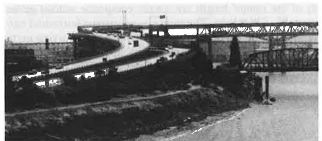
FIGURE 3 Marquam Bridge east approach ramps.
