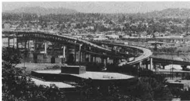
FIGURE 2 Marquam Bridge west approach ramps and main spans.
