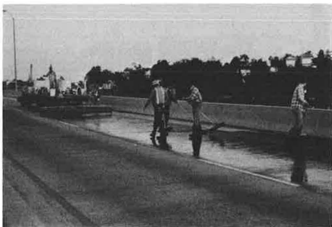
FIGURE 2 Application of HMWM resin.
