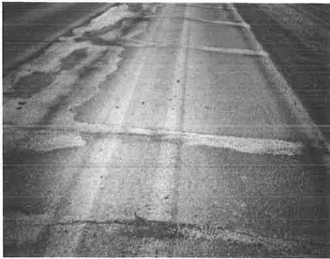
FIGURE 5 Spray patch of cracks with emulsion and sand aggregate—created small ridges at cracks that are detrimental to rideability.
