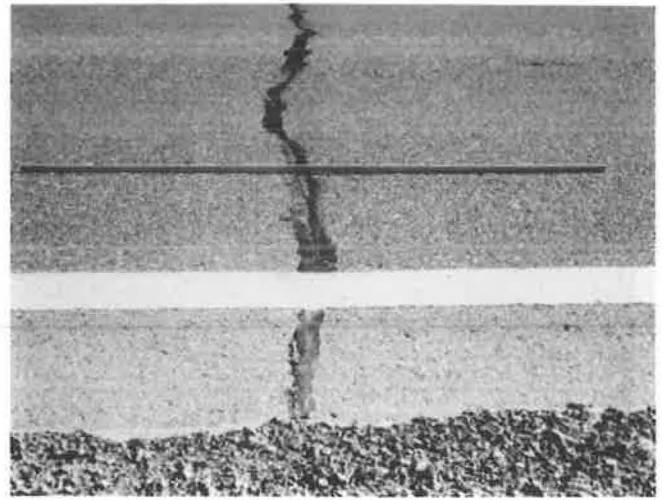
FIGURE 14 Slight cupping of transverse crack on Highway 17, sealed test section with Hydrotech 6160.
