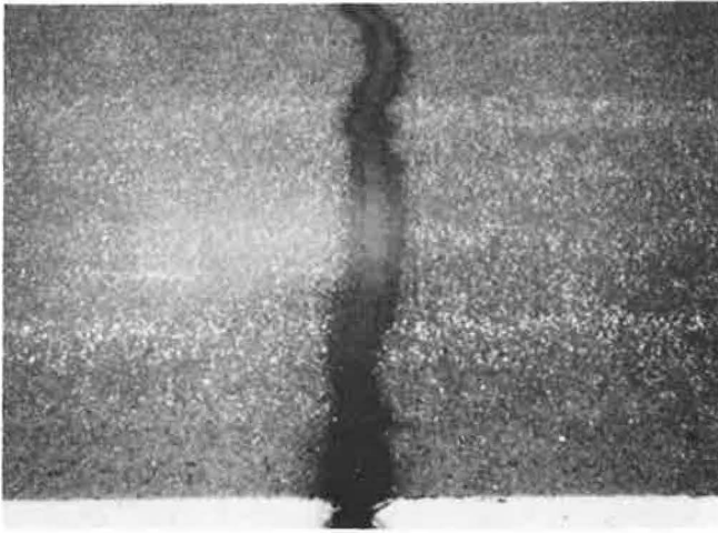
FIGURE 9 Recommended sealant materials overfilled sufficiently to cover edges of routed crack.
