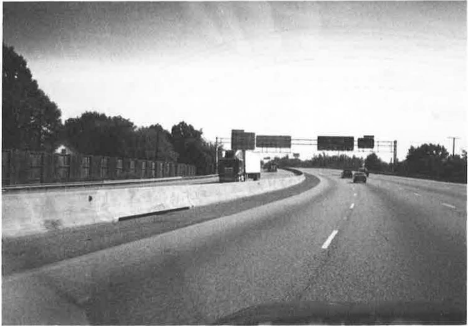
SHIFTED MEDIAN BARRIER—FROM DRIVER'S PERSPECTIVE
