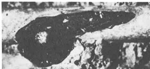
FIGURE 16 Rust filling void in concrete (5).
