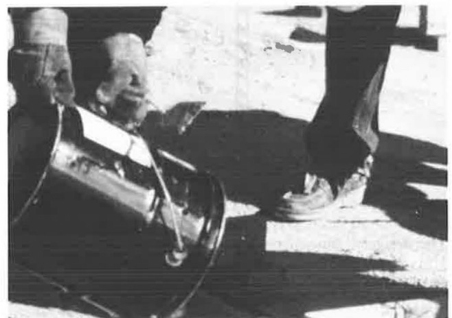
FIGURE 12 Pouring the epoxy mortar through the block-out holes.
