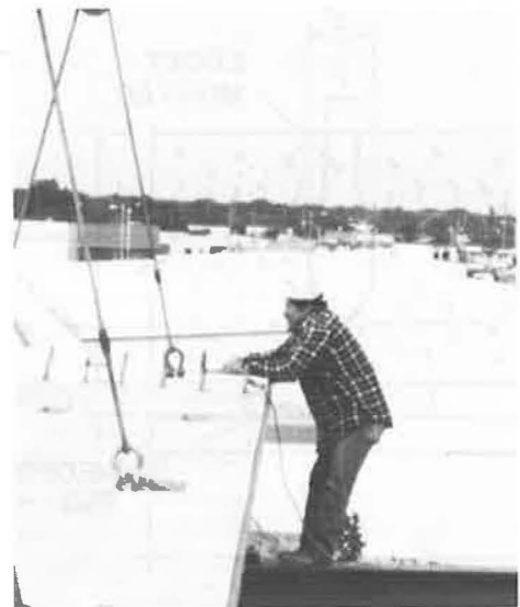
FIGURE 10 View of a panel being placed.
