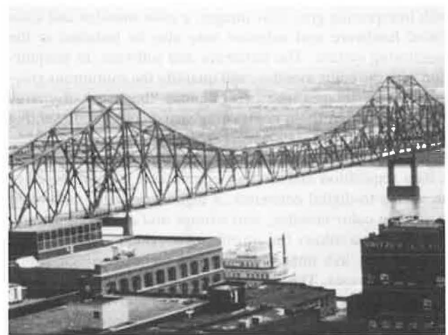
FIGURE 6 Martin Luther King Jr. Memorial Bridge spanning the Mississippi River between St. Louis, Missouri, and East St. Louis, Illinois.
