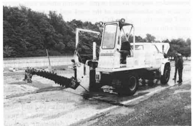
FIGURE 10 Whiphammer used at Aberdeen Proving Ground.
