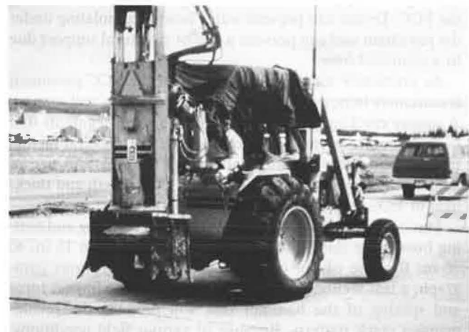
FIGURE 4 Hydraulic impact hammer for cracking PCC slabs.
