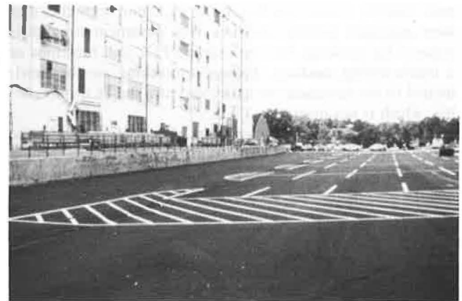
FIGURE 3 Completed asphalt concrete pavement.
