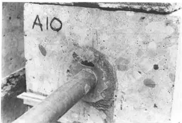
FIGURE 3 Photo of void above dowel anchored using fluid cement grout.
