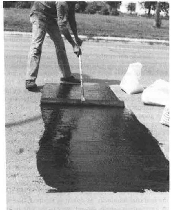
FIGURE 3 Spreading emulsion on test strip.
