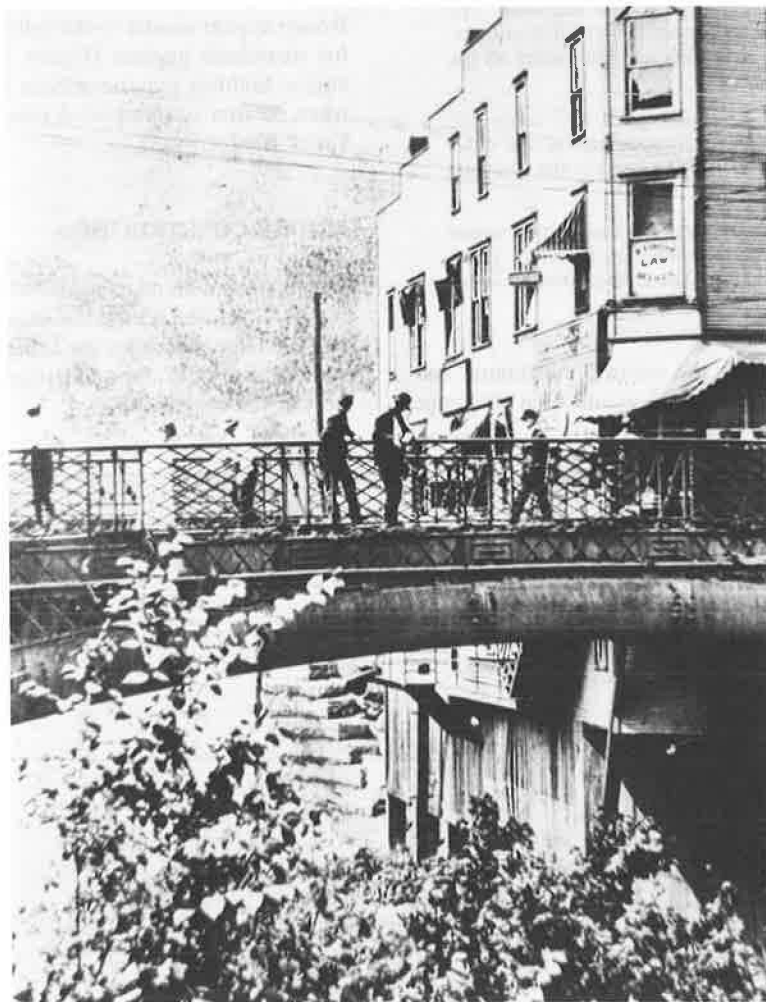
FIGURE 3 Tubular arch segments of the Dunlap's Creek Bridge. Photo courtesy of the Museum of American History, Washington, D.C.
