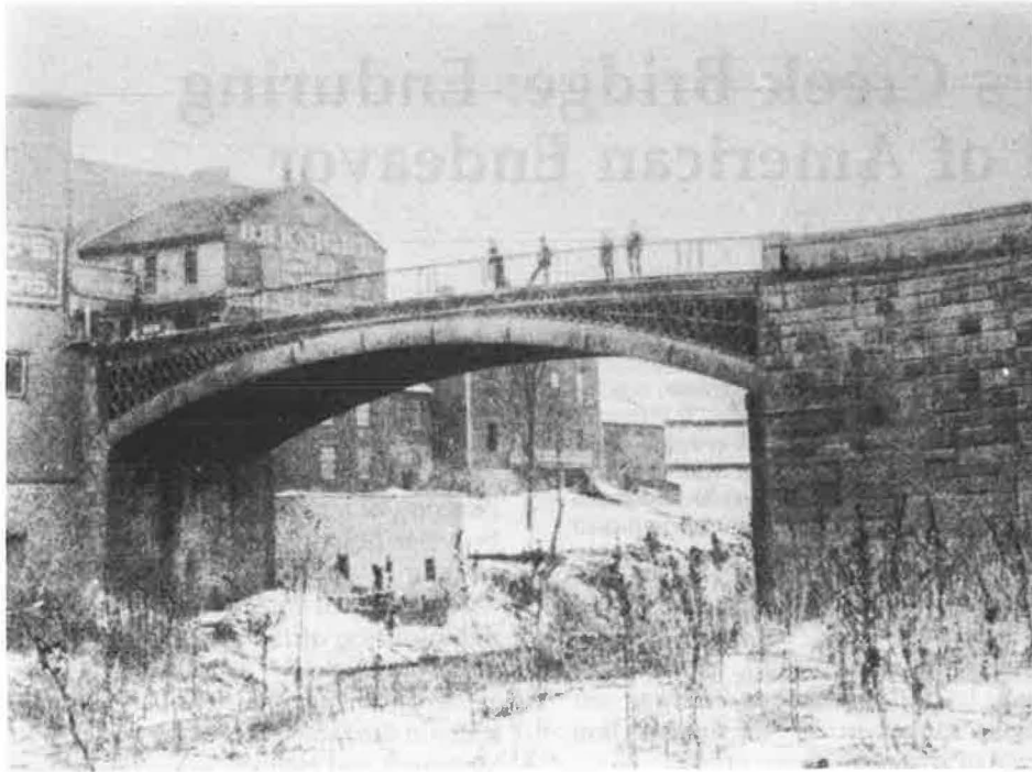
FIGURE 1 The Dunlap's Creek Bridge of Brownsville, Pennsylvania, the first cast iron bridge built in the United States. Photo courtesy of the Prince Maccus Publishing Company.
