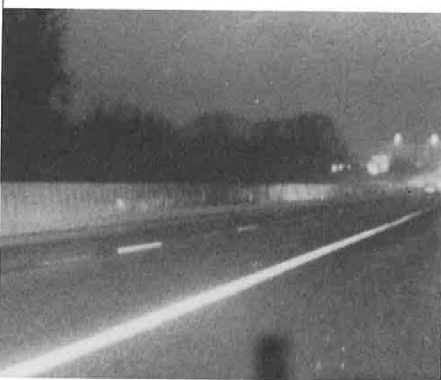
FIGURE 8 Schuylkill Expressway (I-76), Philadelphia, Pennsylvania: large beads in epoxy installed Dec. 1986; standard beads used for skipline between large-bead skips; Dec. 1986 during recovery after rain.
