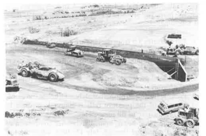
FIGURE 18 Backfill operation at Deep Creek.
