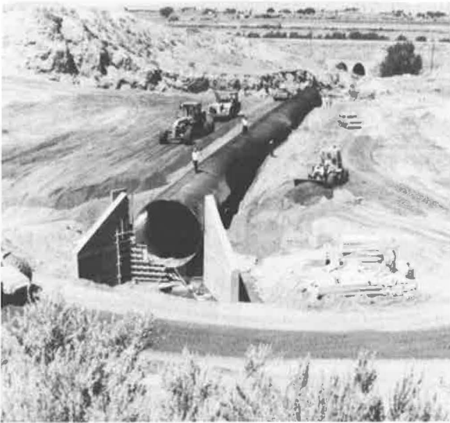
FIGURE 19 Backfill operation at Deep Creek.
