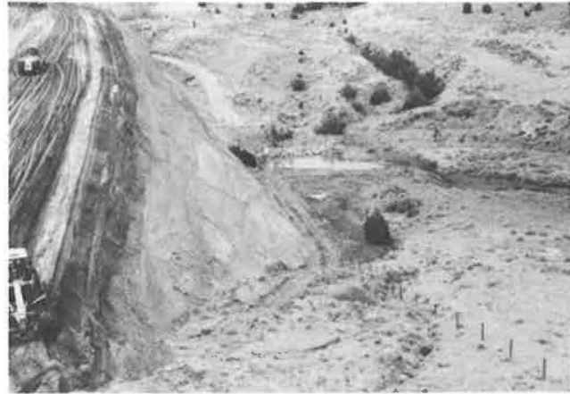
FIGURE 22 Partially completed fill at Spring Creek.
