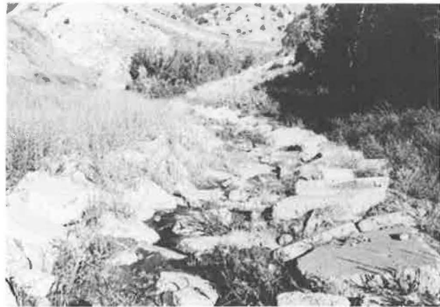
FIGURE 23 Completed fill at Spring Creek.
