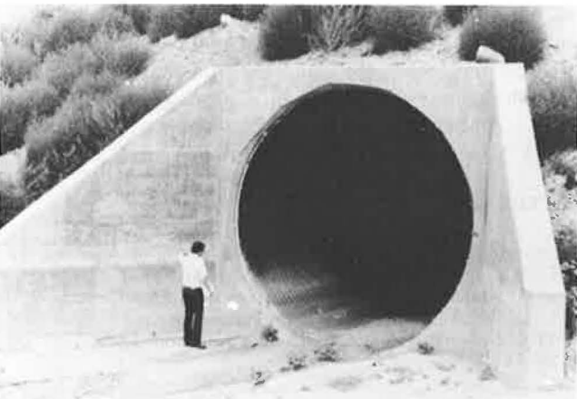
FIGURE 21 Completed inlet headwall and wingwalls at Deep Creek.
