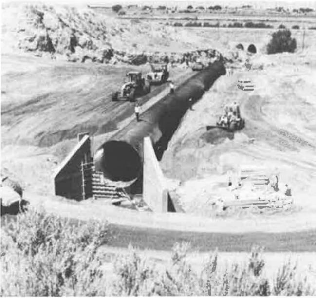
FIGURE 19 Backfill operation at Deep Creek.
