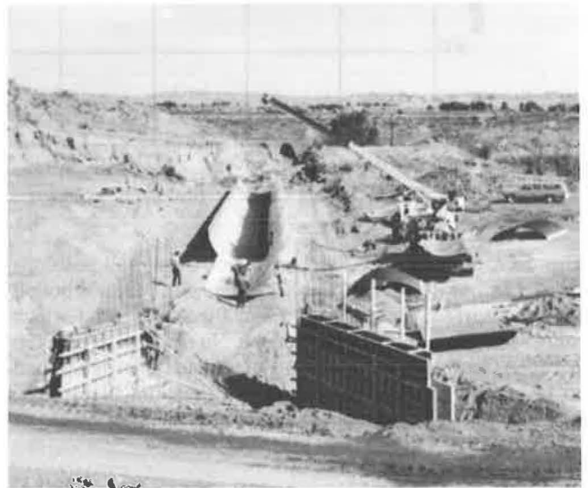
FIGURE 17 Pipe assembly on pre-shaped bed at Deep Creek.
