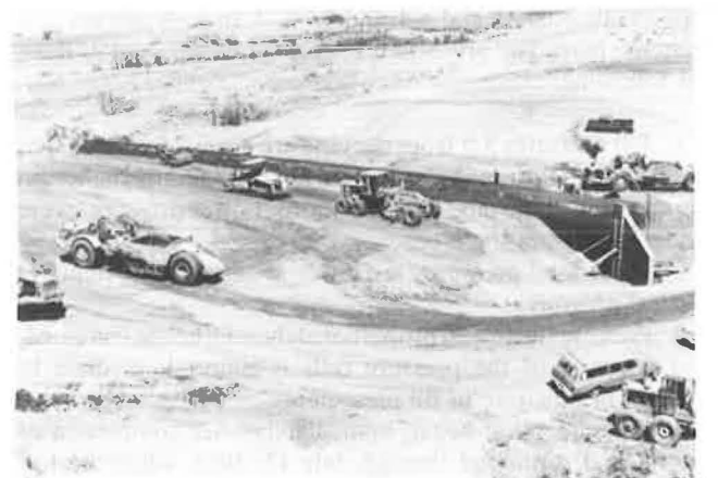
FIGURE 18 Backfill operation at Deep Creek.
