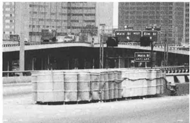
FIGURE 3 Type 2 object marker with supplemental flashing lights.
