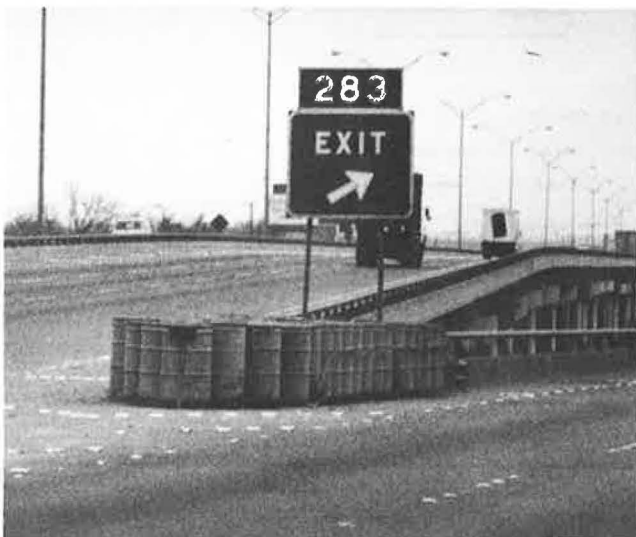
FIGURE 1 Type 2 object marker at front of crash cushion.
