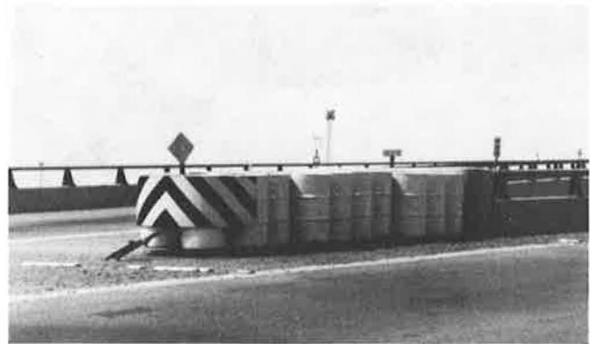
FIGURE 2 Chevron nose panel and type 1 object marker.
