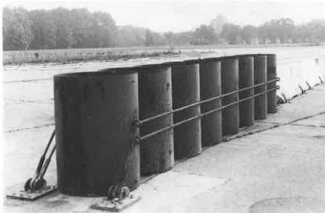
FIGURE 11 Connecticut narrow hazard crash cushion. Cylinder 1 (nose): 1/8 in.; cylinder 2: 3/16 in.; cylinder 3: 1/4 in.; cylinder 4: 1/4 in.; cylinder 5: 1/4 in.; cylinder 6: 5/16 in.; cylinder 7: 3/8 in.; cylinder 8: 1/4 in.
