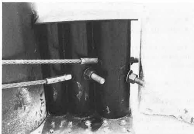
FIGURE 12 Stand-alone concrete-filled steel tubular backup structure.
