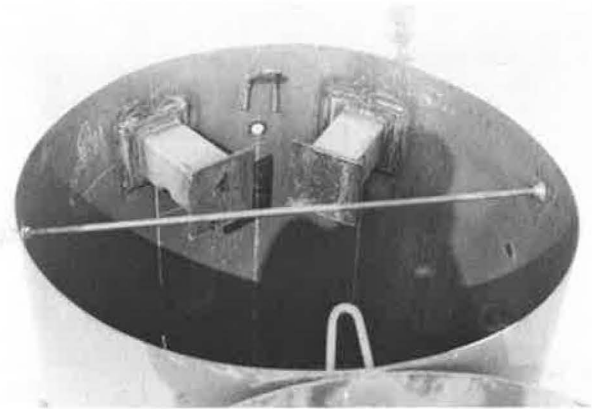
FIGURE 14 Box beam stops and tension rods.
