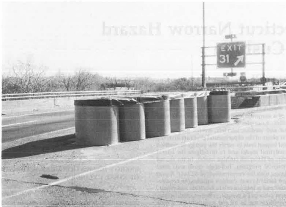
FIGURE 1 The Connecticut Impact Attenuation System (CIAS).
