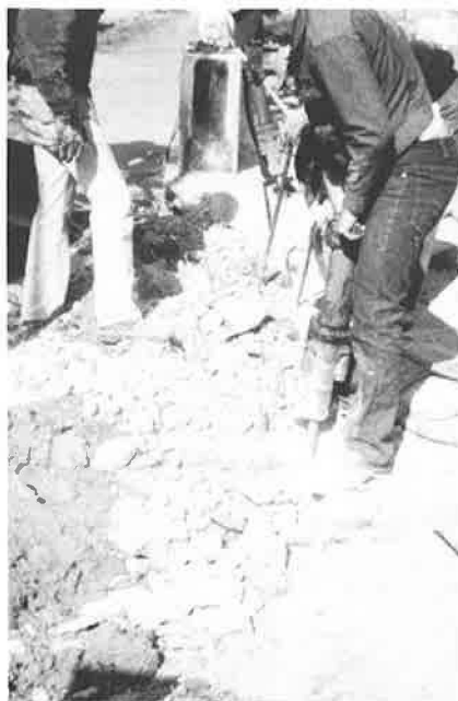
FIGURE 8 Removal of bridge handrail.
