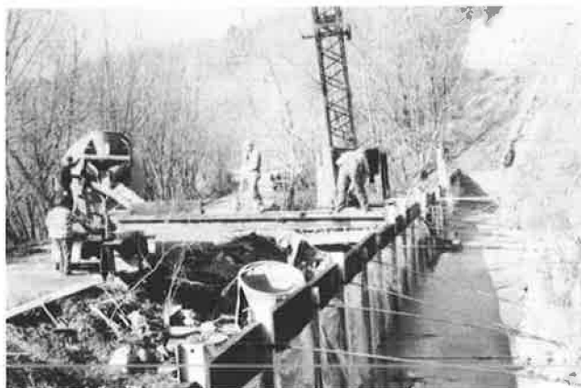
FIGURE 12 Actual placement of flowable mortar.
