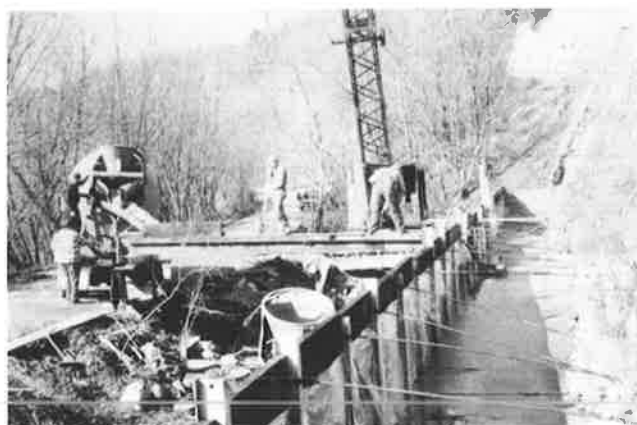
FIGURE 12 Actual placement of flowable mortar.
