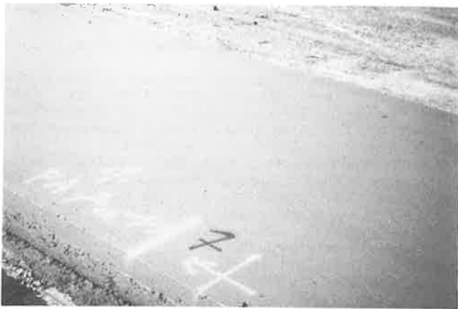
FIGURE 15 Construction of slab. Note sealed appearance of upper surface and straightness of slab edge. Maximum thickness laid was 32 m.
