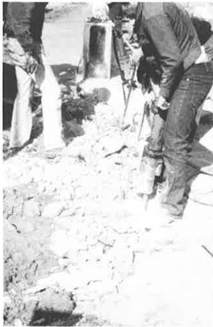
FIGURE 8 Removal of bridge handrail.
