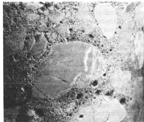
FIGURE 14 A limestone aggregate with preexisting cracks that salt water has moved through. This aggregate would probably deteriorate under freeze-thaw conditions.
