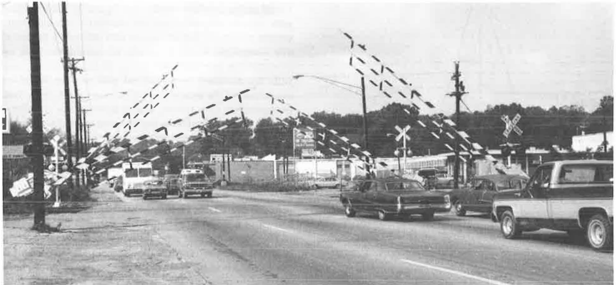
FIGURE 3 Four-quadrant gate system installed at Cherry Street crossing in Knoxville, Tennessee.
