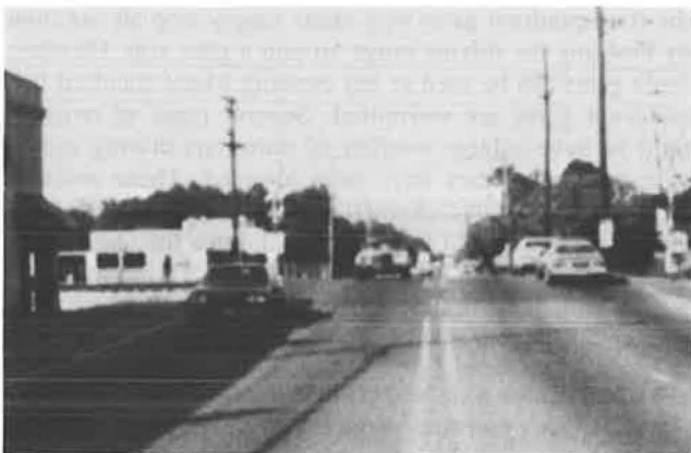
FIGURE 4 Four-lane, undivided roadway crossing.
