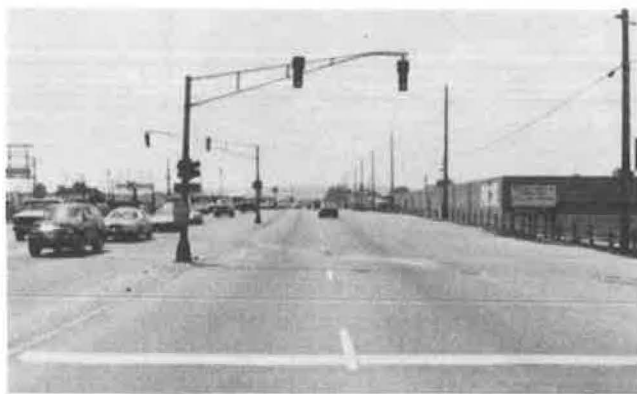
FIGURE 11 Highway traffic signals used at a crossing in Denver, Colorado.
