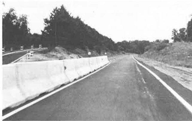
FIGURE 2 Site 1, Route 29, Leon, Virginia.
