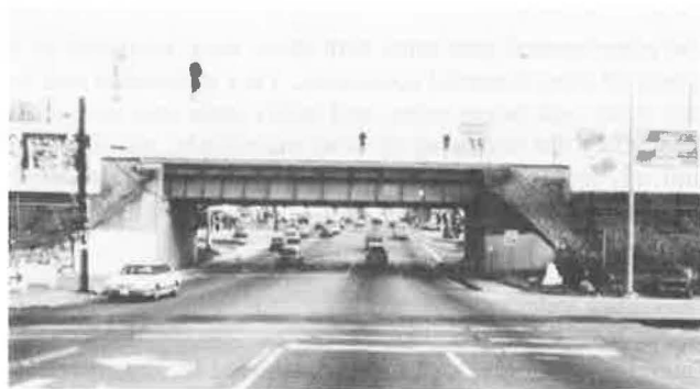
FIGURE 12 Highway traffic signals used at a crossing in Knoxville, Tennessee.
