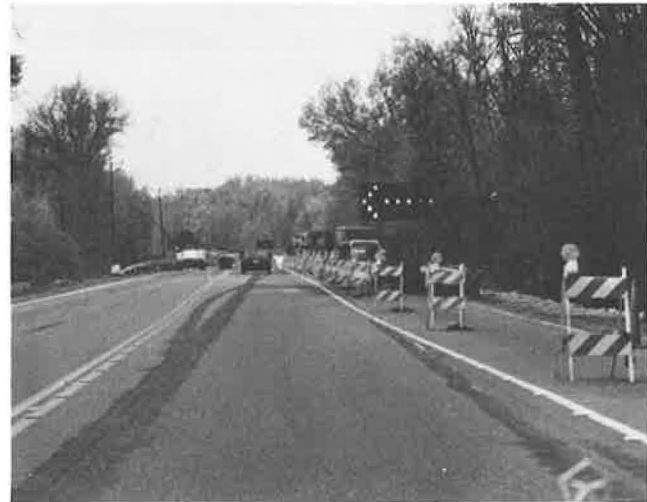
FIGURE 10 Site 2, Route 1, Fredericksburg.
