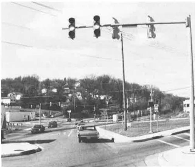
FIGURE 14 Highway traffic signals at crossing with complex roadway geometrics in Knoxville, Tennessee.
