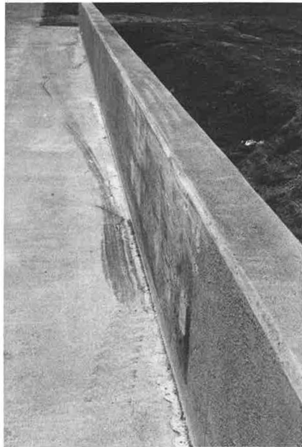
FIGURE 16 Vertical concrete parapet after Test 7069-6.
