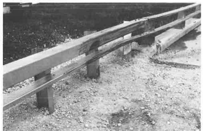
FIGURE 7 Barrier and vehicle damage after Test 0382-1.
