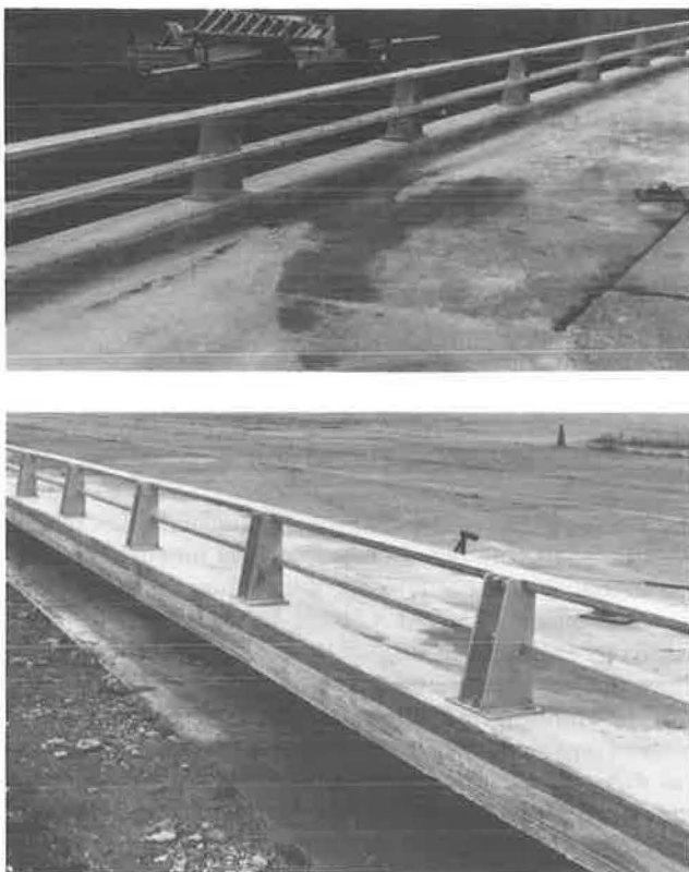
FIGURE 1 Wyoming tube-type bridge rail.
