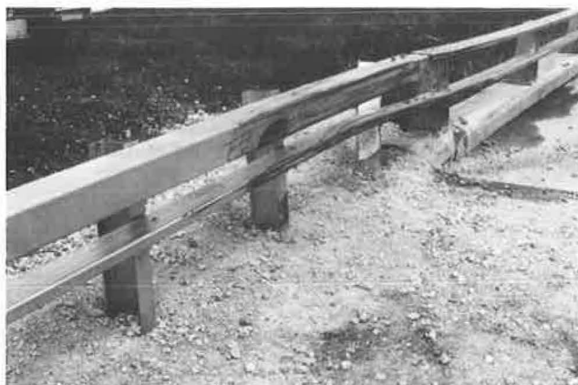
FIGURE 7 Barrier and vehicle damage after Test 0382-1.
