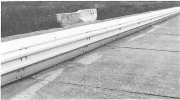
FIGURE 3 MK-9 barrier test installation.
