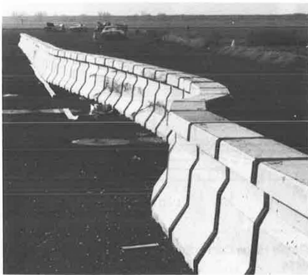
FIGURE 14 Deflected barrier after impact, Test 445.
