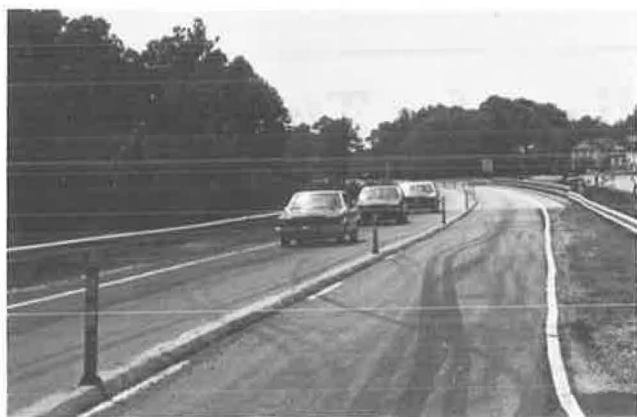
FIGURE 1 Temporary asphalt median.
