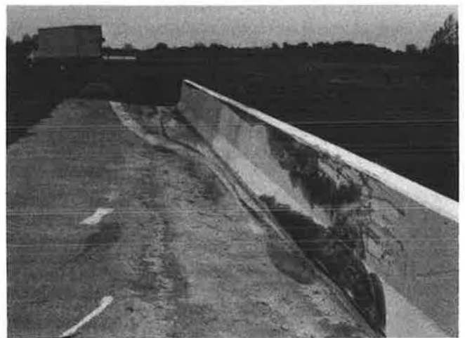
FIGURE 29 Thirty-two-in. F-shape after Test 7069-11.
