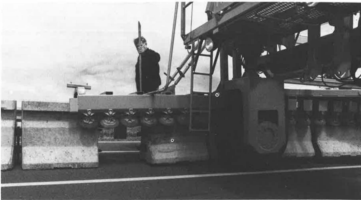
FIGURE 21 Aligning barrier for connecting carried barrier and placed barrier.
