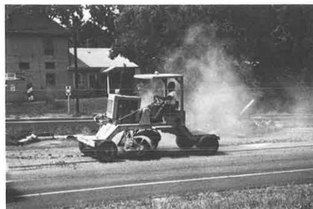
FIGURE 5 Median removal: top , front-end loader removing median; bottom , sweeping loose gravel.
