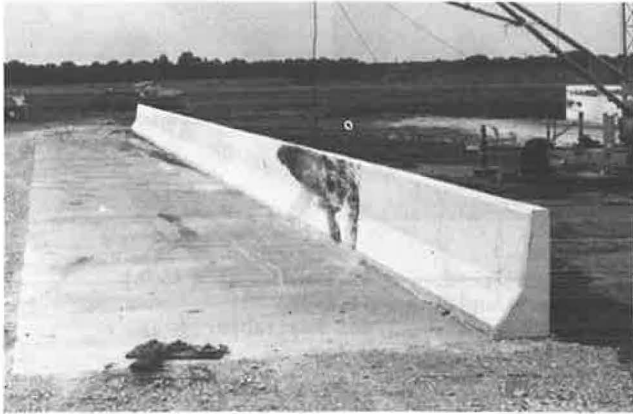
FIGURE 32 Thirty-two-in. safety shape railing after Test 7069-14.
