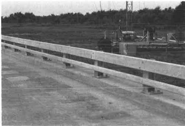
FIGURE 2 Prototype test installation of Illinois 2399-1 railing.
