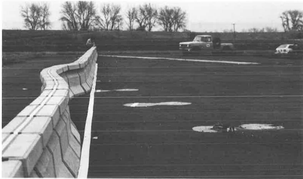
FIGURE 10 Car and barrier after impact, Test 444.
