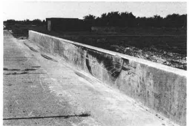
FIGURE 19 Thirty-two-in. vertical parapet after Test 7069-16.
