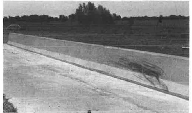
FIGURE 23 Thirty-two-in. F-shape after Test 7069-3.
