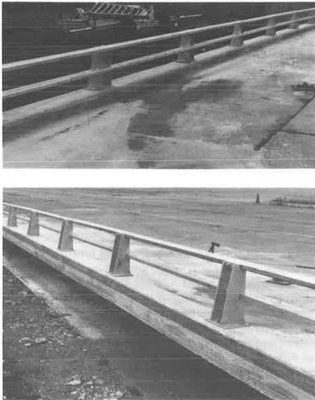
FIGURE 1 Wyoming tube-type bridge rail.
