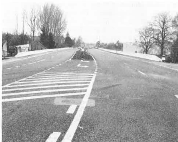
FIGURE 4 Porous asphalt sections on N 56 Ath–Ostriches at Ath.
