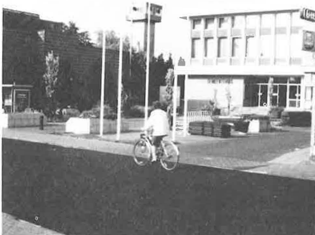
FIGURE 5 Porous asphalt sections on city streets at Kurne.
