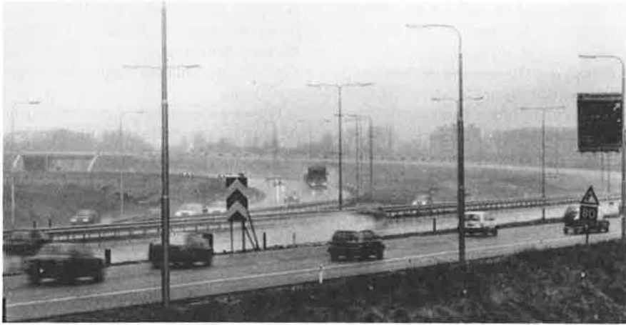
FIGURE 7 Visual improvements stemming from the use of porous asphalt.
