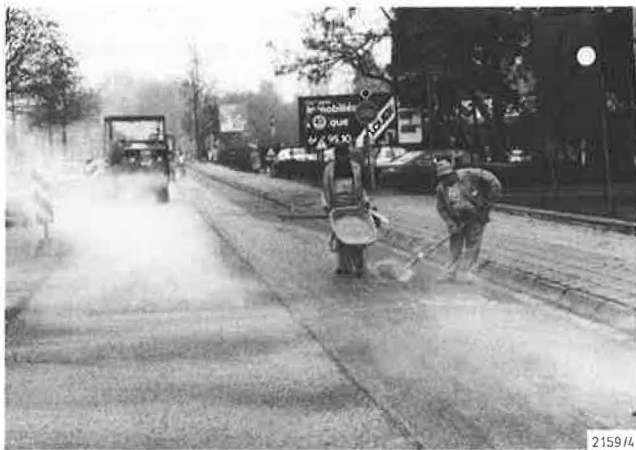
FIGURE 9 Spreading filler on a newly laid porous asphalt surface.
