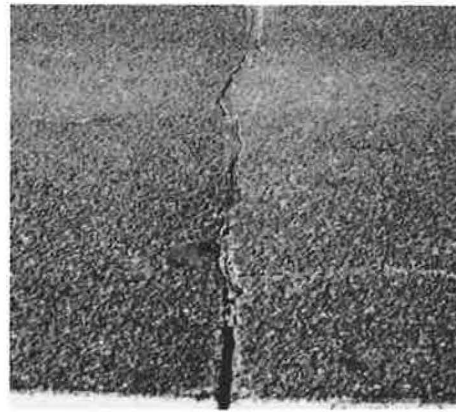
FIGURE 12 19- × 19-mm rout and seal with Meadow 164R Test Section 7, 1981 (February, 1989).
