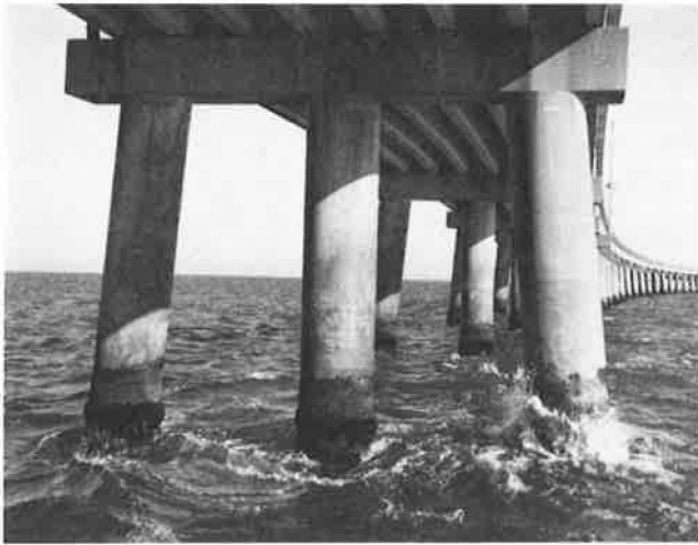
FIGURE 1 General view of facility.
